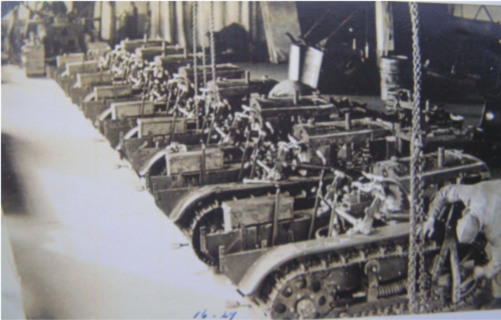
8 Trail Tractors being built in the Portland Shops
