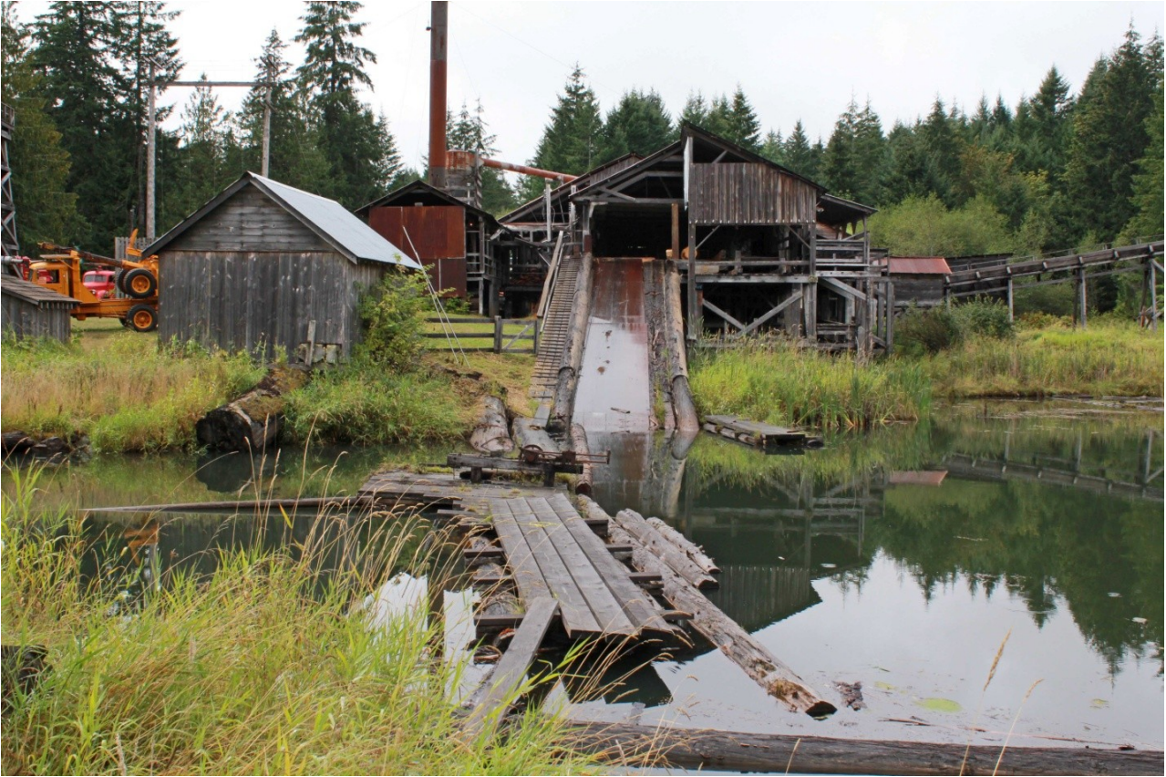
Figure 1: Log Pond & Jack Ladder – McLean Sawmill. Dan Seaberg, used with kind permission.
