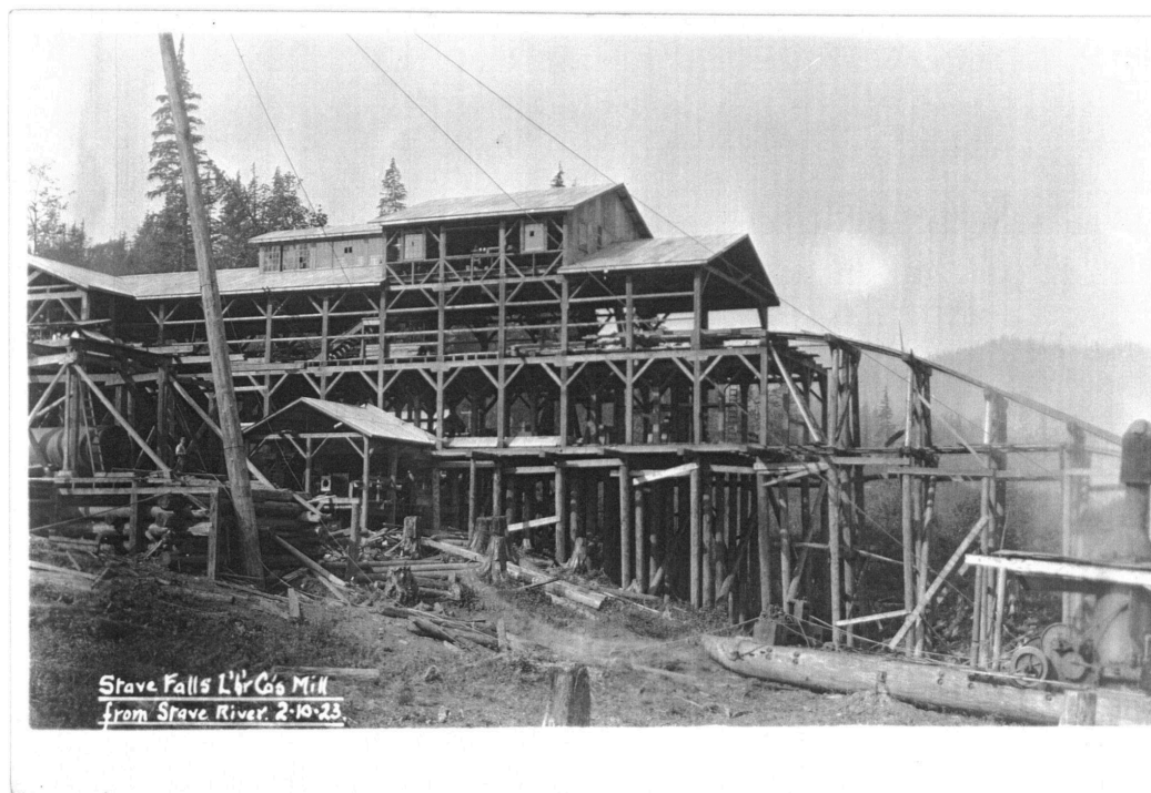
Figure 3: Stave Falls Lumber Company mill under construction circa 1923. Prominent are the heavy clear timbers used in the construction and the steam donkey in the foreground. Photographer unknown. Author's collection.
