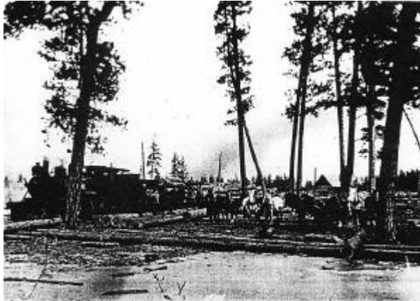
Decking and loading teams and the Kettle Valley Railway, Coquihalla Valley.
